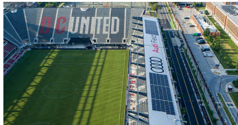
SOLAR PANELS LINE THE ROOF OF AUDI FIELD (WARD 6)
